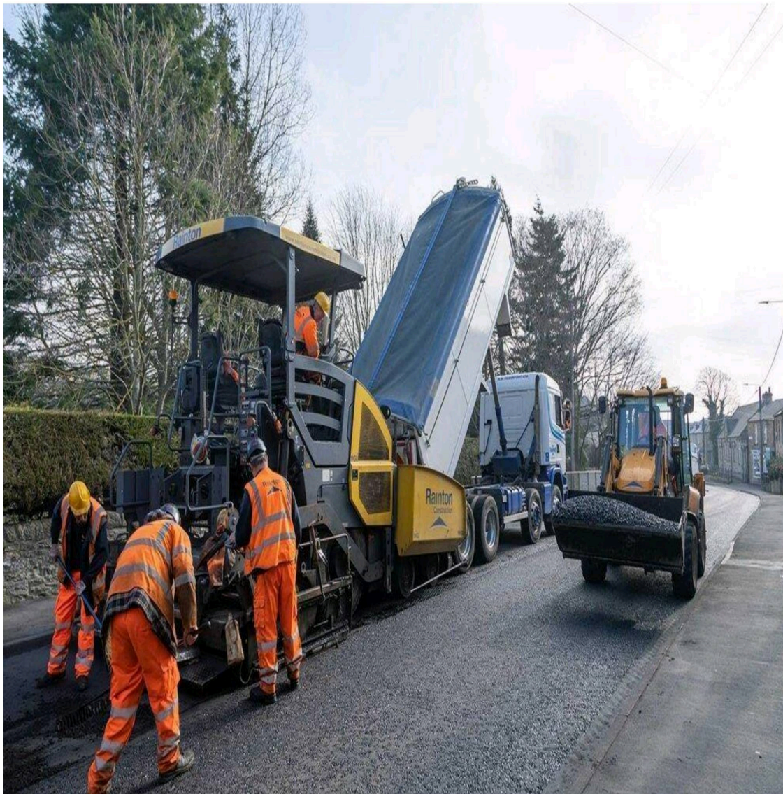
construction of roads by using plastic waste
